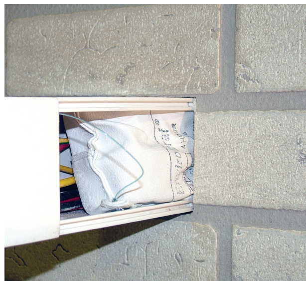
Figure 3.2b Intumescent pillow within non-flame propagating trunking
