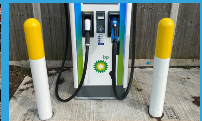
A barrier around a public rapid chargepoint
