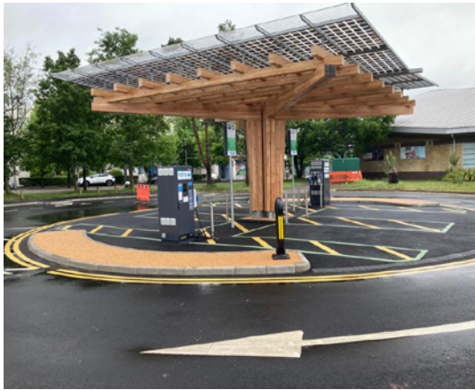
Chargepoints with local microgeneration and storage.
