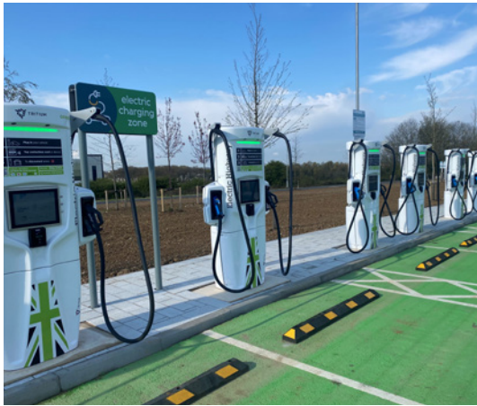
350kW chargers at a motorway service station.
